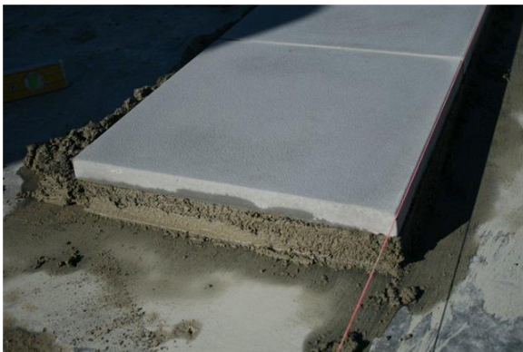
Ideal mortar mix
