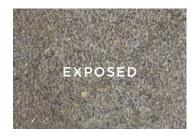
A textured finish where the top 2-3mm of aggregate is revealed, creating a slip resistant finish.
