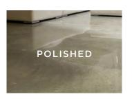
A finish where the surface is not honed and no exposure of aggregates is seen. The floor is polished to a glossy finish.
