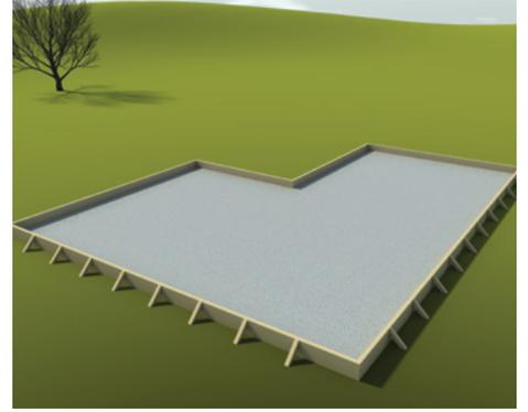
**3** Within this boxed area, a Jacking slab is poured to a height of 180mm\* using a specifically engineered seismic resilient Firth concrete mix. [\*Sizes may change depending on the specific solution designed for your site.]
