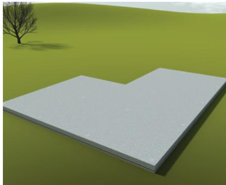
**8** Once cured, boxing is removed to reveal a twin-slab floor.
