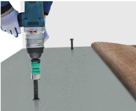
**2** Using a standard rattle gun, they insert and screw high tensile threaded bolts into the various RaftJack™ points raising the upper slab up off the lower slab until the upper slab (and house) is level.
