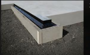
HotEdge<sup>®</sup> and HotEdge Extra<sup>®</sup> panels are temporarily fixed inside the perimeter of the form work, prior to concrete pour.
