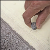
60mm tornado wire screw connectors are placed at 300mm centres alternating top and bottom to provide regular fixed anchor points into the concrete slab.
