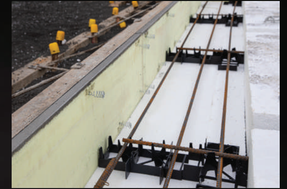
1 HotEdge® and HotEdge Extra® panels are temporarily fixed inside the perimeter of the form work, prior to concrete pour. NOTE: Tornado screws anchor the panels into the slab.
