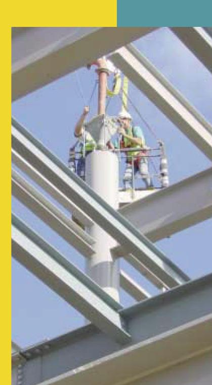
Firth Self Compacting Concrete (SCC) is concrete that flows into place under its own weight, without segregation and flow blockage. SCC can flow through congested reinforcement or complex formwork and achieve complete filling and consolidation with minimal mechanical compaction, and thus saves time, labour, equipment requirements and formwork damage; and it does all this silently. What's more, the off the form finish can be exceptional, reducing rework and saving time.
