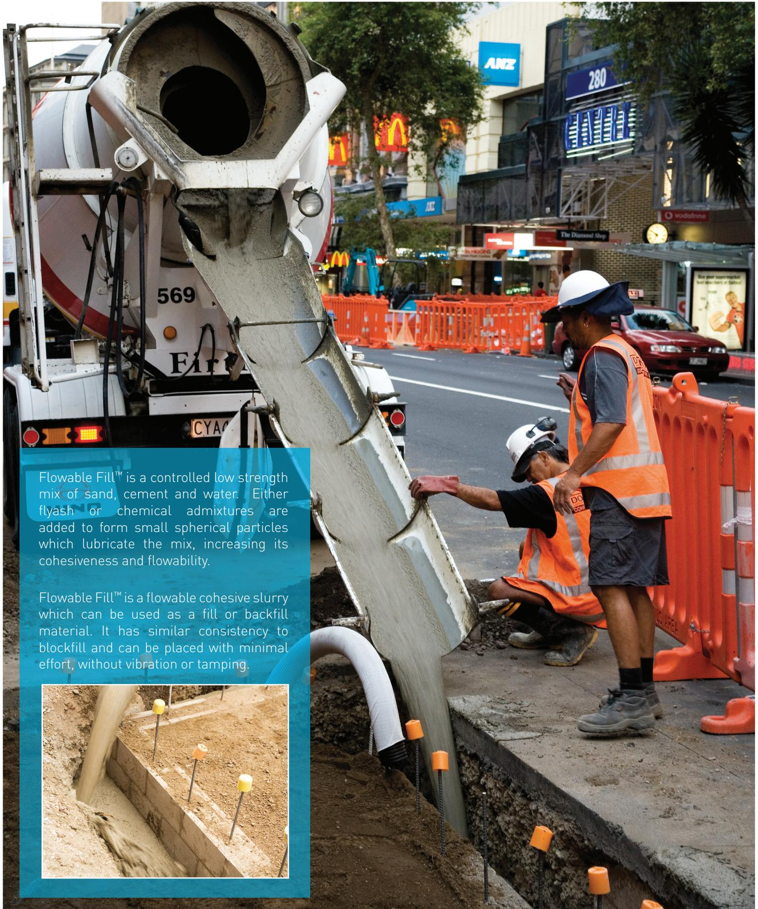
Flowable Fill™ is a controlled low strength mix of sand, cement and water. Either flyash or chemical admixtures are added to form small spherical particles which lubricate the mix, increasing its cohesiveness and flowability.
