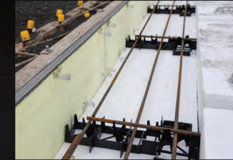
1 HotEdge® and HotEdge Extra® panels are temporarily fixed inside the perimeter of the form work, prior to concrete pour.
