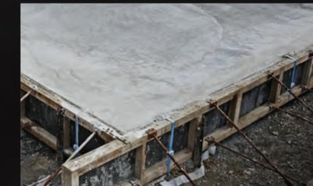
2 RibRaft RaftMix® concrete is poured level with the form work leaving the top of the HotEdge Extra® panel uncovered. The HotEdge® panels for brick cladding should be positioned 25mm below the rebate former to create a ledge covering the beveled top of the panel to support brick veneers.
