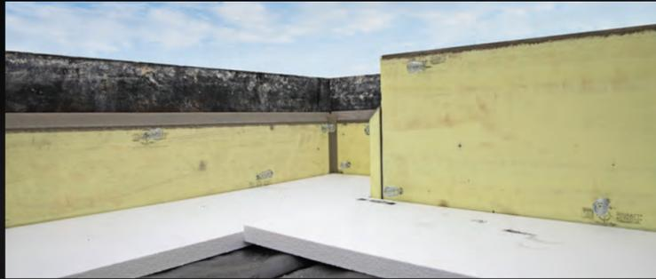
HotEdge Extra® has the same slab integration and durable finish as HotEdge® but has been specifically developed to improve the thermal envelope of buildings using alternative cladding systems to brick veneers.
