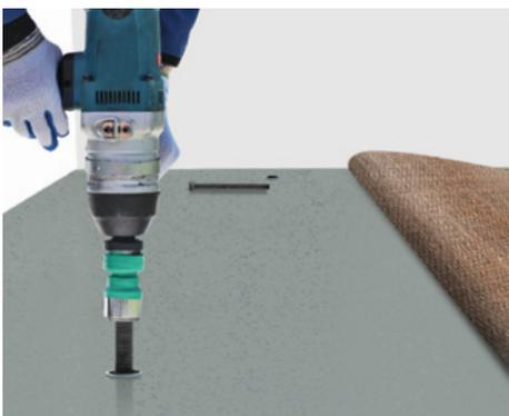
**5** When cured, the RaftJack™ bolts are simply removed by unscrewing them. The jack point holes covered and floor covering relaid.
