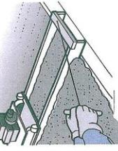
**11** FOR SMALL JOB SLABS UP TO 100mm THICK A HAND TAMPER MAY BE USED.
