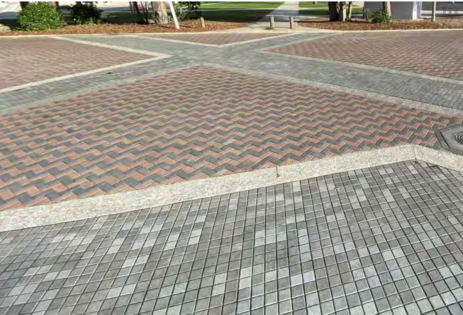
Above: Holland Set - Black Sands & Natural (both Bush Hammered) and Piazza 80mm - bespoke mix design (Honed) Below: Holland - Black Sands & Terracotta (both Fair Faced) and Holland Sett - Black Sands (Fair Faced, Honed & Bush Hammered)
