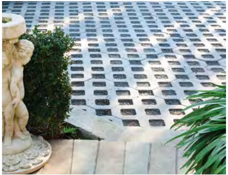
Grass Paver - Natural (note: image shows paver before grass has established)
