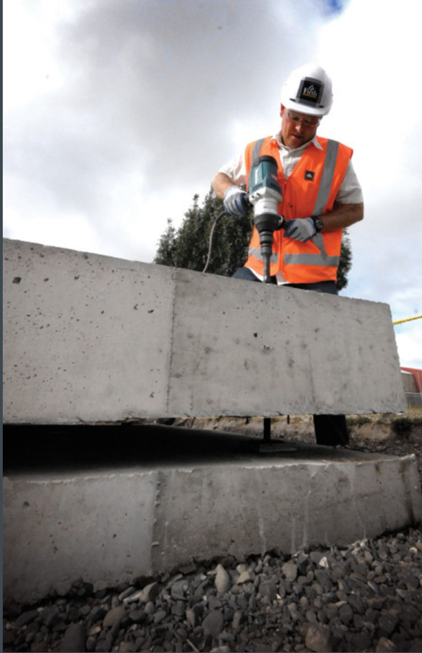
FIRTH PROTOTYPE RIBRAFT® TC3 SLAB IN TESTING
