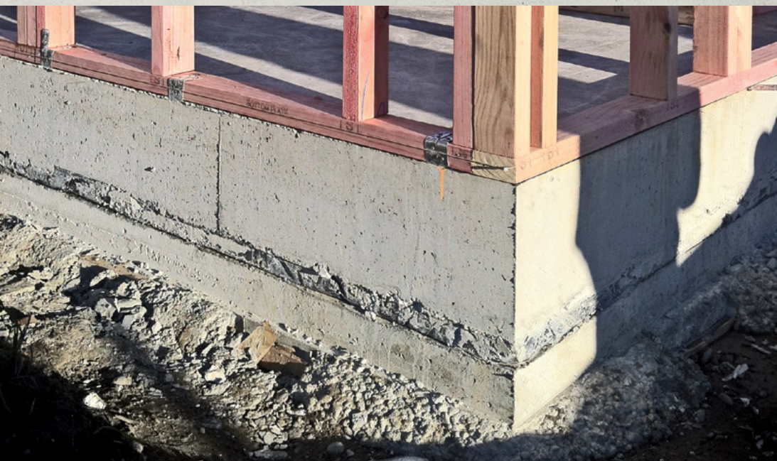
TC3 SLAB ON NEW BUILDING
